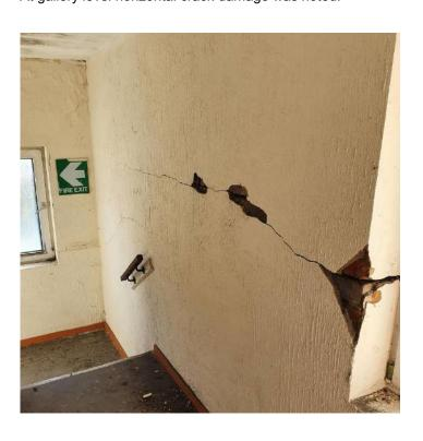
Front Left Stairwell At first floor level a single 203UB section spans to the front wall and supports a section of the floor slab above. No evidence of corrosion was noted to the steelwork. The steel does not appear to have any fire protection. Diagonal cracking is visible on the inner leaf of the front wall where the steel is bearing on to it. On the internal west wall face at ceiling level horizontal crack damage was noted running the full length of
