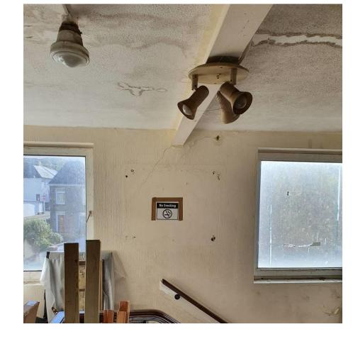
The walls appear to have some superficial crack damage and there is evidence of damp on some wall projections.
